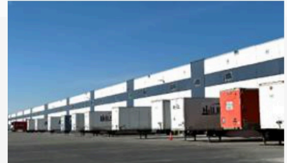
Multi-tenant – Council Bluffs, IA
