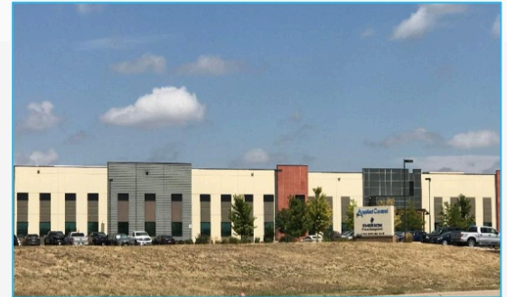
Applied Control Equipment – Denver, CO
